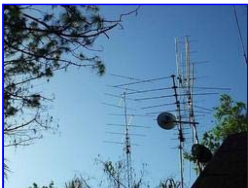
ANTENNAS USED DIRECTIVE SYSTEMS 2M-2304 AND A PROCOMM 10GIG DISH, IN THE BACK GROUND IS THE 6M ARRAY
