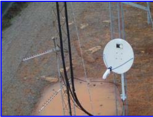
Top: 2.4ghz Internet Links Bottom: 1.2ghz ATV Link
