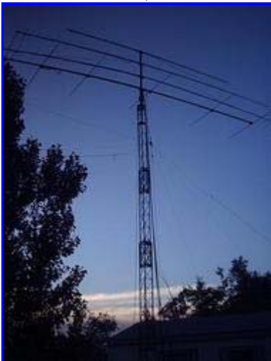
K7XC - Main Tower. 50 Mhz - 6 ele K7XC HB on 30' Boom at 39'. 144 Mhz - M2 18XXX on 33' Boom at 41'. 222 Mhz - M2 7WL on 31' Boom at 43'. 432 Mhz - 9WL K1FO on 27' Boom at 45'.
