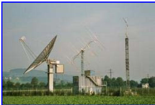
The impressive antennas at HB9Q club station: 50 foot dish for 432 and 1296 MHz plus 8 x 19 elements for 144 MHz
