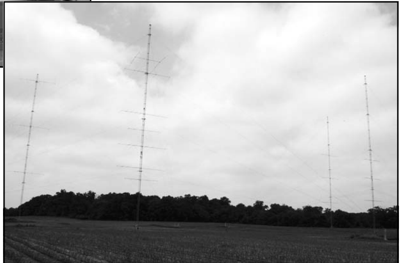
Figures 4 and 5—The new station and antennas at John, N3HBX's, contest station in Poolesville, MD. The station has four 190 foot rotating towers with stacks on 40–10 meters. In the shack there are two SO2R operating positions. See N3HBX's two-part series in the November/December 2005 and January/February 2006 issues of NCJ for more details on this contest station. Mark KD4D and John entered as a multi-single using KD4D. Mark did CW and John worked phone. John notes that looking at the scores of those who beat them indicates that they spent too much time on phone and too little time on 10 meters. However, he says they had a lot of fun and nothing broke! Their score put them in 4th place in the W/VE M/S category.
