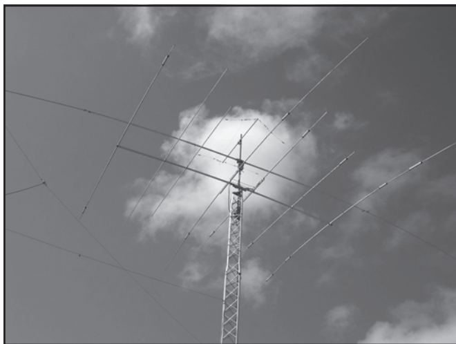
The HAM-let's main tower with the tribander and 80-meter dipole.
