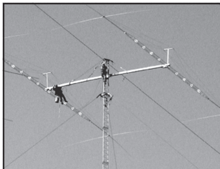
Matt, KC1XX, and assistant Andrew (no call) tuning up the 80-meter Force 12 Yagi (185 feet in the air).
