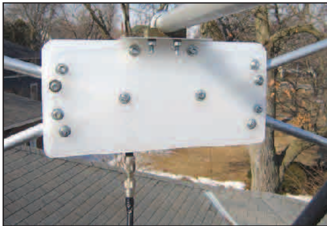
Figure 3 — Close-up of the back side of the modified cutting board used as a center support and insulator.
