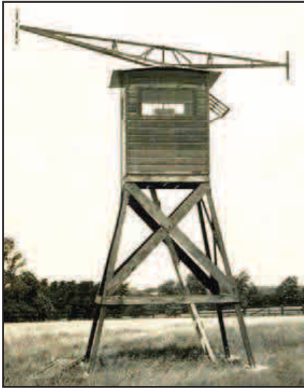
One of eight Adcock Direction Finders (DFs) in the Hawaiian Islands. These helped pilots find their way from the Mainland to the Islands. The DFs each used Hallicrafters SX-28 receivers.
