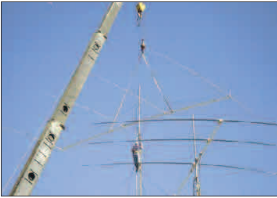
Field Day at W6SON, with four towers and antennas for 3.5 through 432 MHz, including 4 elements on 40 meters!
