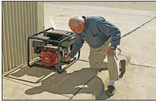
Ralph Brown, KA5KVF, is shown setting up the generator at the Garland Emergency Communications Center. Their ARES/RACES team simulated a severe ice storm that created havoc to communications and the city's electrical power grid.
