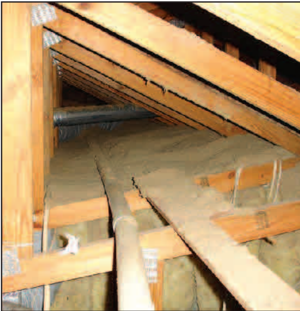
Figure 4 — The ac conduit parallels the antenna elements.
