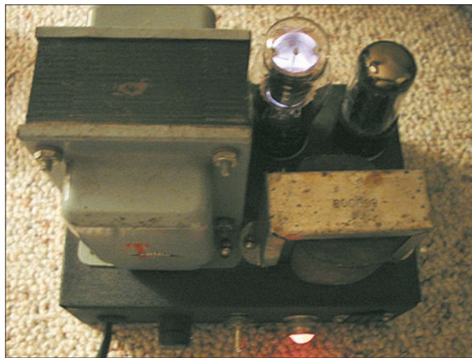
Figure 4 — The power supply repaired and fired up after 50 years.
