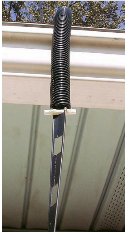
Figure 3 — The split tubing installed on the ladder-line with the plastic pen stop in place.
