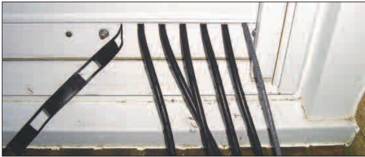
Figure 4 — A view from outside.
