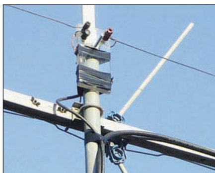
Figure 5 — Loop center insulator mounted on mast as described in text.
