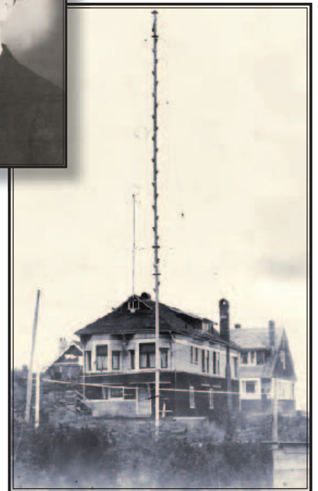
Antenna is an inverted L type consisting of a cage 75 feet long and 63 feet high for the top part, with a lead-in 45 feet long. A counterpoise of 12 wires 85 feet long and fanned somewhat is located directly beneath the antenna.
