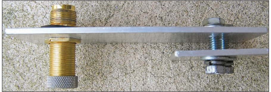
Figure 5 — Side view of assembled antenna mount.
