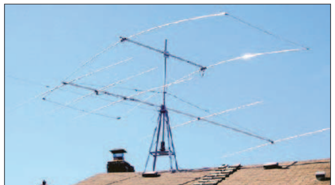
Figure 10 — Moxon mounted on the HF roof tower above the five element 10 meter beam. The roof ladder shown helps save the shingles and enhances safety.
