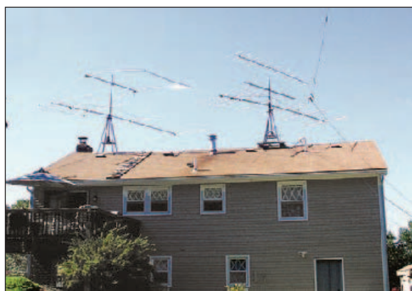
Figure 11 — The two roof towers, with my VHF antennas to the right: K1FO 2 meter, 2 meter FM and seven element homebrew 6 meter Yagi.
