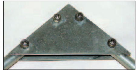
Figure 6 — Detail of the corner construction showing the two triangular plates and locking hex nuts. For an explanation of why the hardware looks new and the aluminum looks old, see the discussion about mechanical performance.
