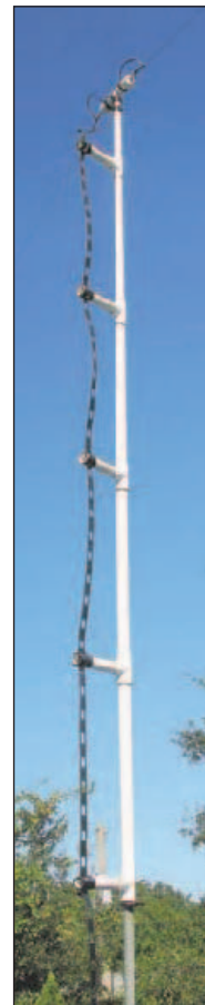
Figure 5 — The complete PVC support mounted on the mast.
