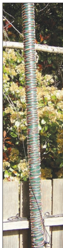
Figure 12 — Latest version of 160 meter vertical. Installed and neighbor friendly.
