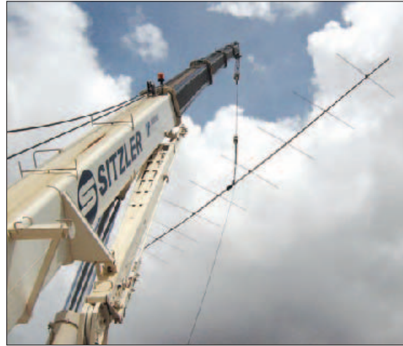
Figure 1 — How's this for a "skyhook"? David, VK2CZ, operated as VK8AA in Australia's Northern Territories with this monster beam. The antenna was 85 feet long and it was 140 feet in the air, thanks to the crane.
