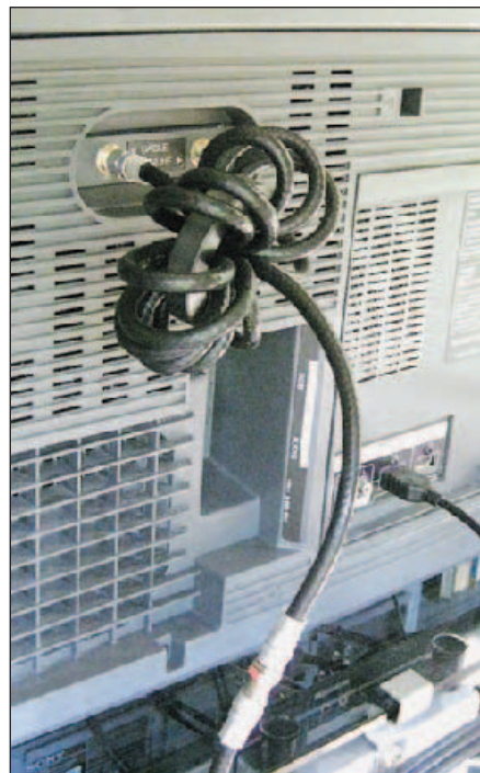
Figure 3 — The common mode choke installed on the coax input to the TV. This helped, but wasn't the final answer.
