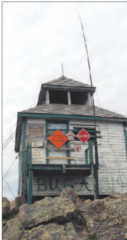
The abandoned fire observation hut on the summit. Note the steel guy cables to prevent the hut from being blown off the mountain and my antenna mast flexing in the wind.
