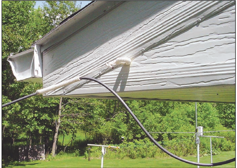
Figure 1 — RG-8X coax anchored to the author's house.
