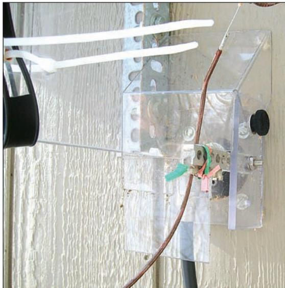
**Figure 8** — Entry point for a single coax cable. The removable "greenhouse" cover is made from a single piece of 0.063 inch thick material bent to shape in a sheet metal bending brake. A single black thumb screw holds the cover to the threaded base.
