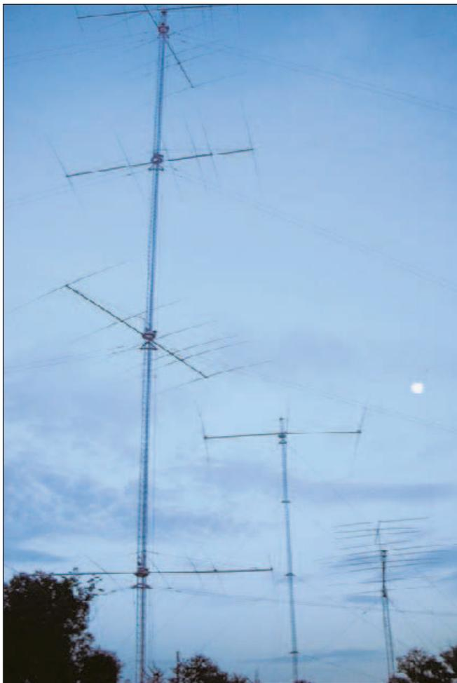
Figure 1 — The moon sets over four stacked 20 meter beams and a 3 element 80 meter beam — and this is only part of the NR5M antenna farm.
