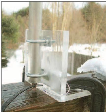
**Figure 1 — View of antenna support L bracket antenna mount made from 0.50 inch thick material. The two 0.25 inch holes in the base section are for potential use with bolts and nuts.**
