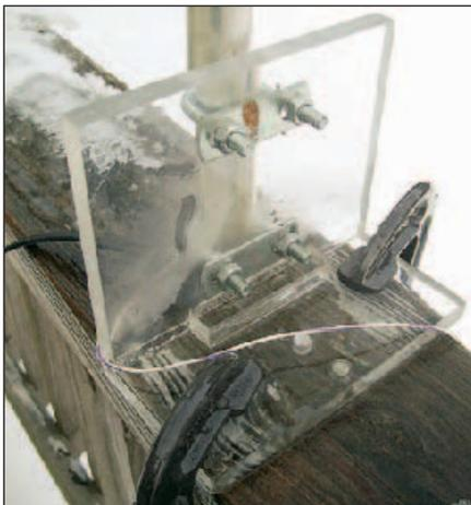
**Figure 2 — Another view of the L bracket. Note the 0.50 inch square cross section reinforcing brace glued to the inside corner of the upright section/horizontal base. This was added after the mount had been in successful service for some time, as insurance against high winds.**
