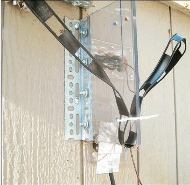
**Figure 6** — Flat vertical antenna support bolted to garage wall with slotted angle steel stock. Without any additional support of any kind, not even guys, this 0.50 inch thick mount previously supported a 23 foot long aluminum homebrew vertical antenna for several years in all sorts of Northeast weather. It's presently serving much lighter duty as a feed line anchor point.
