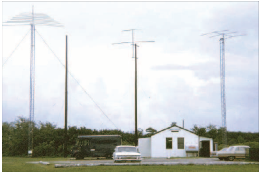
Langley AFB MARS station, a ham's dream antenna farm. From left: Log periodic, dipole mast, VHF antennas and a triband beam.
