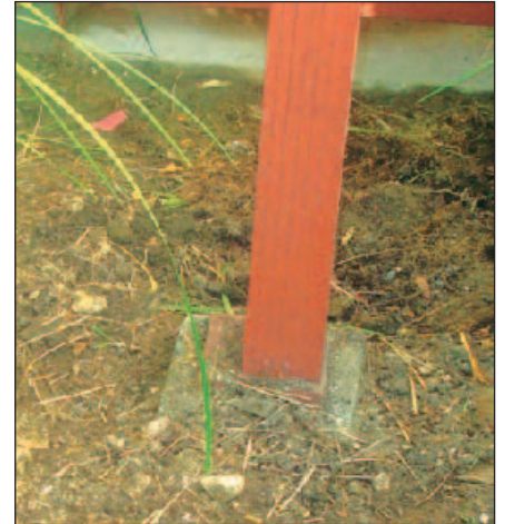
Figure 6 — Finished surface over ground system with top soil covering plastic sheets.
