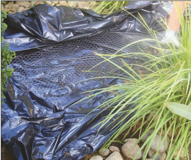
Figure 5 — The screen mesh is triple-wrapped in weed barrier plastic sheets, and covered with a 1 inch layer of top soil for concealment. The mesh is secured in the concrete patio area by double layers of aluminum aircraft aviation tape.
