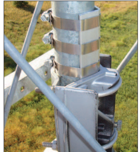
Figure 2 — The completed mounting arrangement has the corner of the aluminum angle ground down to fit into the corner of the rotator bracket. The three stainless steel hose clamps secure the aluminum angle to the mast.
