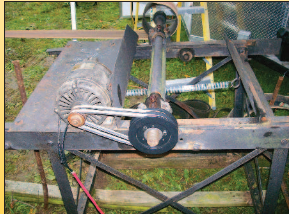
Our 12 V generator setup. The steam engine drive belt is in the rear.
