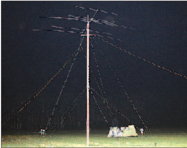
WRTC runs during the 24 hour IARU HF Championships. The contest began at 1200 UTC (4 PM Moscow Summer Time) on Saturday, July 10. The WRTC 2010 Organizing Committee supplied each team with a 20/15/10 meter tri-band antenna on a 12 meter tower, as well as a 40 and 80 meter inverted V dipoles.
