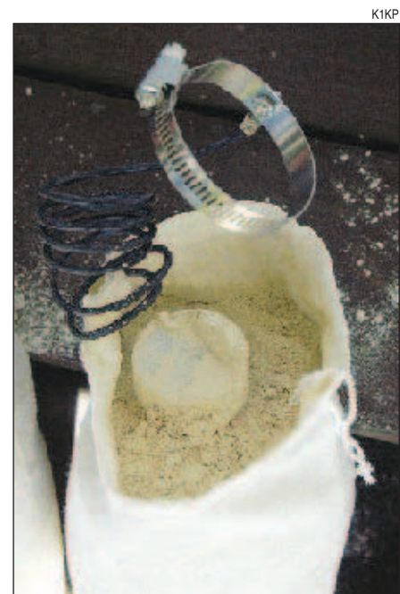
Figure 5 — Bag filled with backfill material and magnesium electrode before closing.
