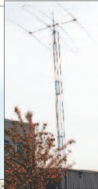
The finished remote location with the tower and beam.
