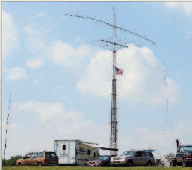
Impressive: The Delaware Amateur Radio Association, DELARA, in Delaware, Ohio, used the Delaware County EMA/911 command post as one of our stations. The tower is a surplus 100 foot crank-up with an older tribander and a homebrew 40 meter dipole. Several wire antennas were strung from the tower as well. We operated using the club call sign, K8ES, as 4A Ohio. Another station was set up using the Radnor Volunteer Fire Department Operations Trailer, also on loan for the weekend. — Stan Broadway, N8BHL
