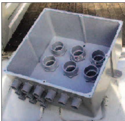
Figure 2 — The box with all adapters mounted.
