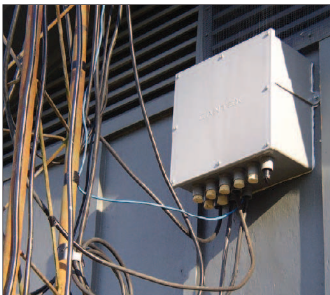
Figure 5 — Box closed prior to wires being dressed to the tower.
