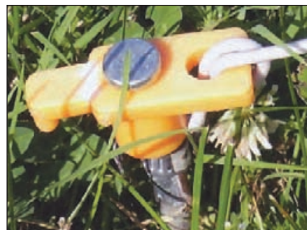
Figure 2 — Close-up of one of the tent stakes. Remember to remove the insulation before clamping the end of the wire to the stake to aid grounding.
