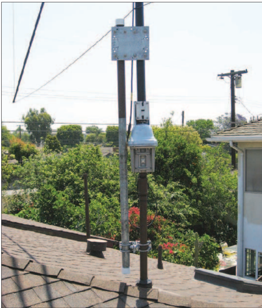
Figure 4 — The rotator to mast clamp plate and U bolts installed finger tight.
