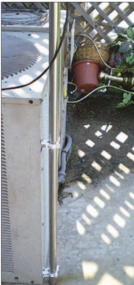
Figure 3 — The two garden-tool clamps are mounted using existing holes and screws on the air conditioning unit. The 2 meter mast is clearly visible.
