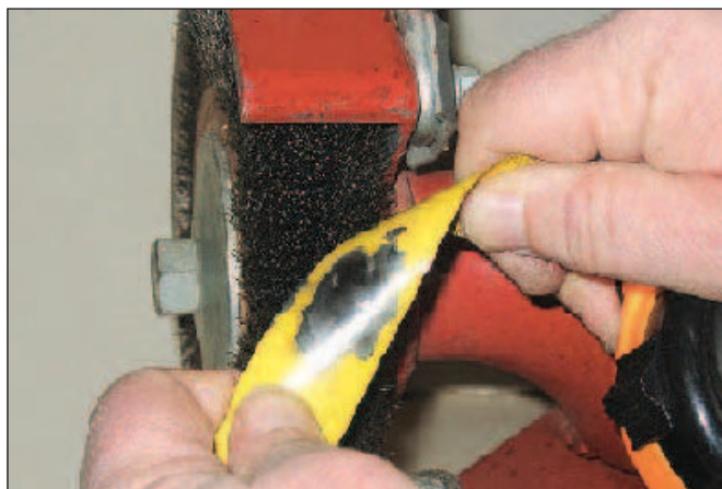
Figure 3 — Bare metal area exposed after paint removal.
