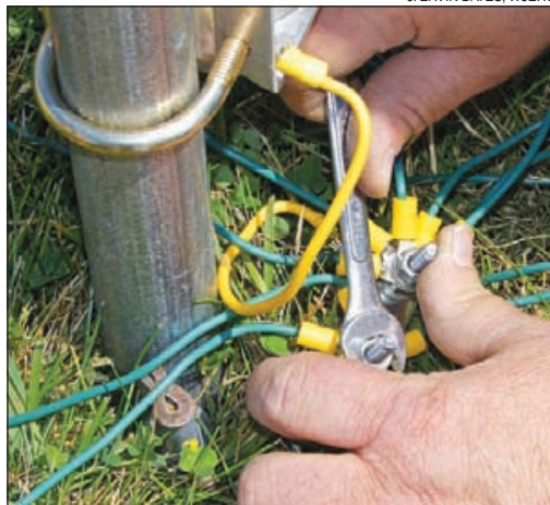
Figure 10 — Connecting the tape measure radial wires to a 3/8 inch U bolt at base of trap vertical.
