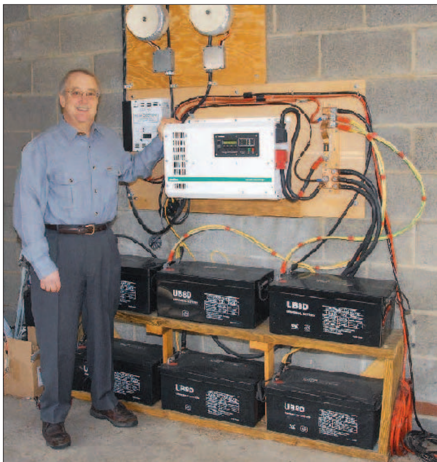
Figure 4 — System along the garage wall. It does not interfere with using the garage for a car. Note the 2 × 4 platform for the batteries. A movable ramp facilitates battery replacement.
