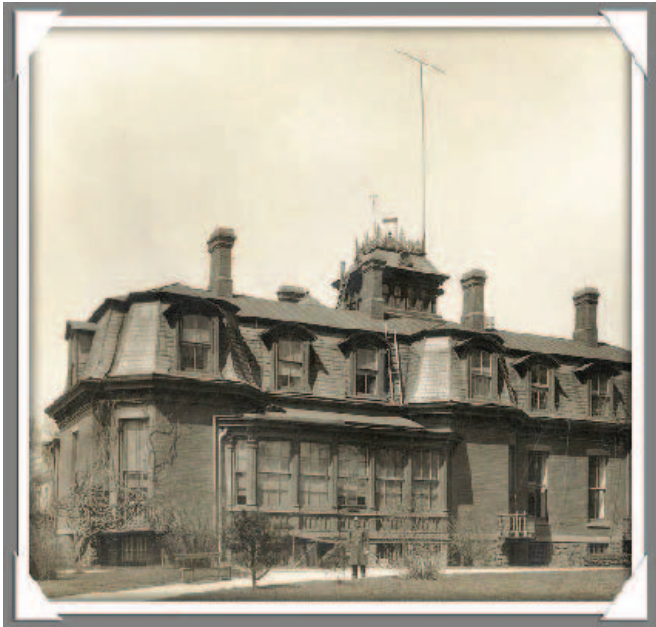
Brooklyn Children's Museum. New antenna on museum building composed of 5 wires, 1½ feet apart, 250 feet long and about 85 feet from the ground. Antenna designed and erected by Frank Hart and others during 1907-1908.
