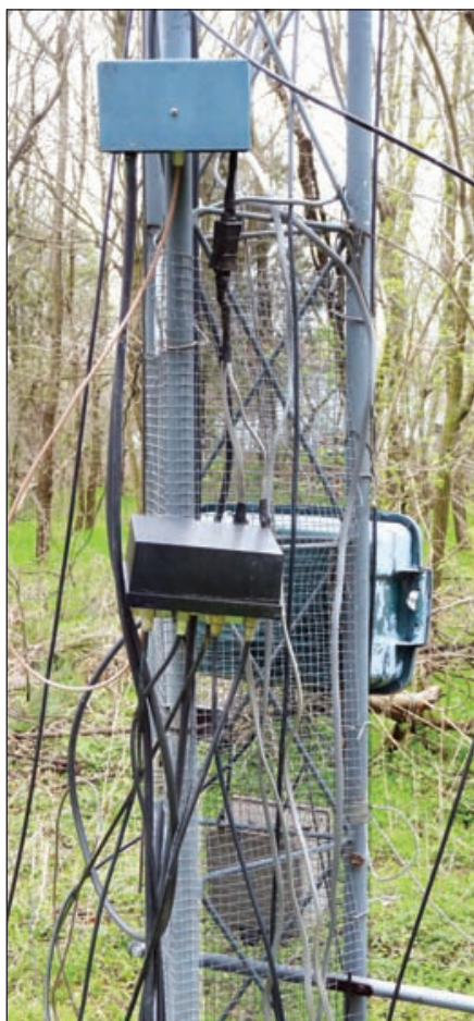
Figure 5 — The RCS-10 remote relay box, mounted on my tower.
