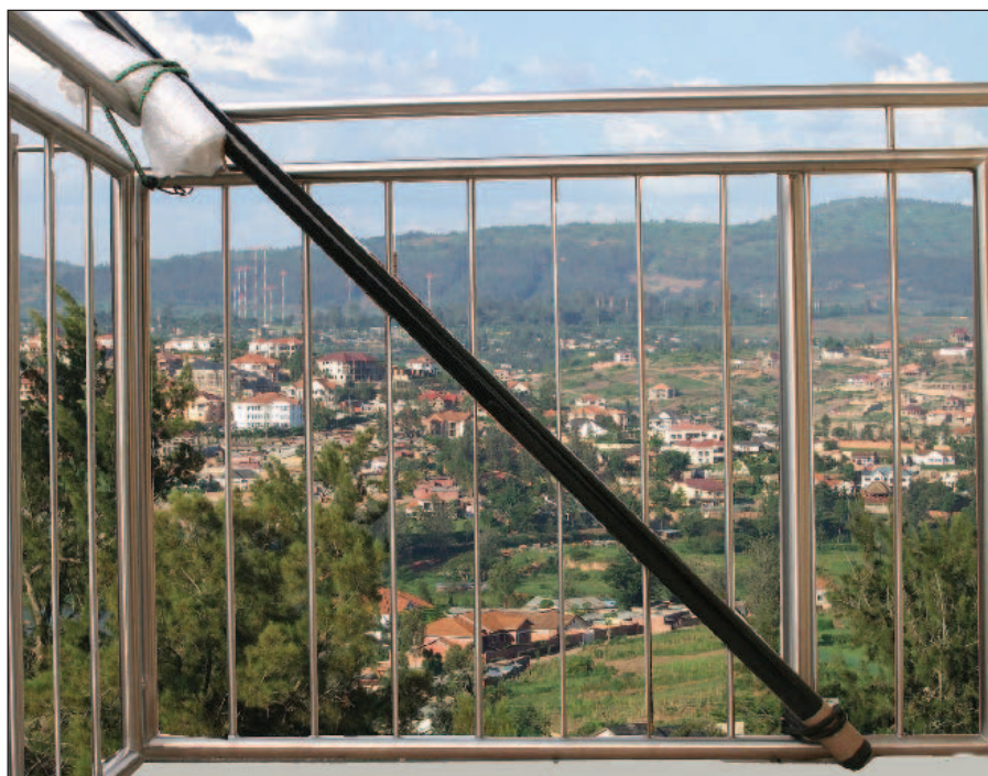
Figure 3 — Details of balcony attachment. Adjustable locking straps are used to secure both the bottom of the pole and the fulcrum on the balcony rail.
