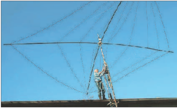
Figure 3 — The Spiderbeam is a two element Yagi with bent wire elements supported by fiberglass spreaders ( www.spiderbeam.com ). Another stressed wire multiband Yagi is the Hexbeam. First offered by Traffic ( www.hexbeam.com ), versions are now also available from others.
