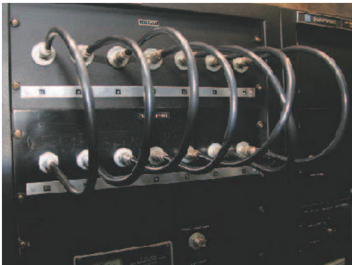
Figure 2 — The patch panel at W1AW is used to interconnect transceivers (bottom row) and antennas (top row) without the need for switches.
