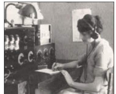
Mrs Paulie Raser, XYL, operating "3CS" 1 kW spark set, remote controlled in cellar, 1923. Receivers from left, long wave, and Paragon RA-6 short wave.
