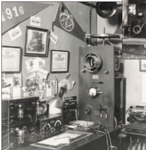
Half-kilowatt spark transmitter "3CS" from 1919 to 1922, equipment is all home built, called it "Big Bertha," receiver is regenerative 150-700 meters with Moorhead Audion Detector and 2 stage amplifier. Commercial marble base key and Baldwin phones.
