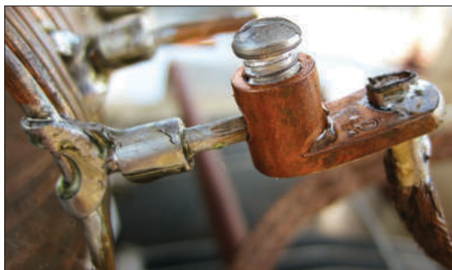
Figure 9 — Final tap assembly showing the ring lug, the #10 AWG wire stub, the copper terminal lug soldered to the ferrule, and the braid jumper.
