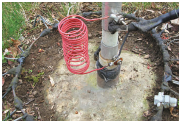
Figure 4 — Feed-line connections, such as on this ground mounted vertical antenna, require protection from the adverse effects of weather. The use of stainless steel hardware and protective tapes can minimize problems.
