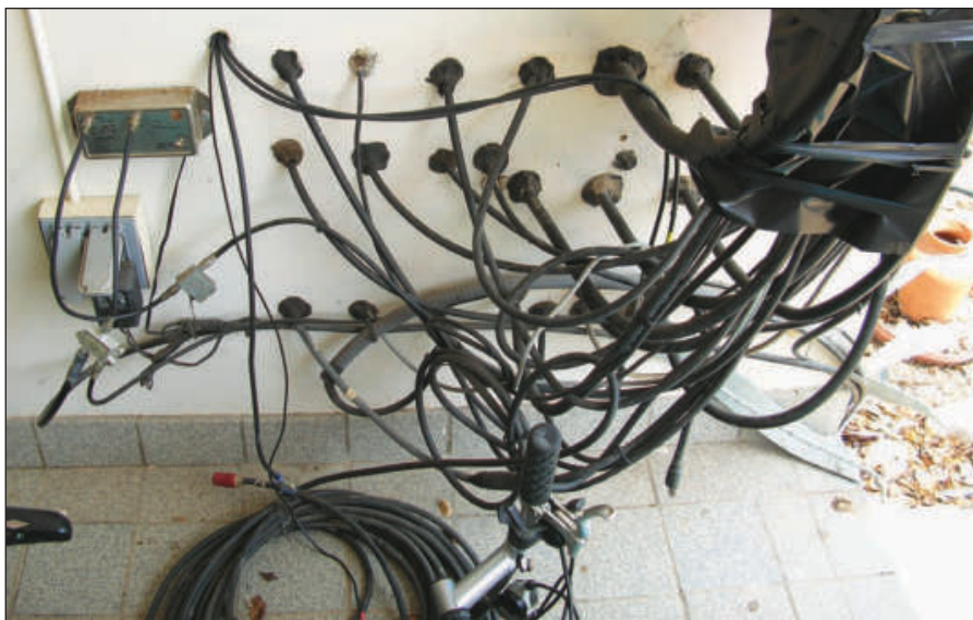
Figure 3 — Multiple transmission lines, such as these at the PJ2T contest station in Curaçao, require multiple connections, multiplying the probability of something failing. Care in installation and frequent inspection will minimize problems.
