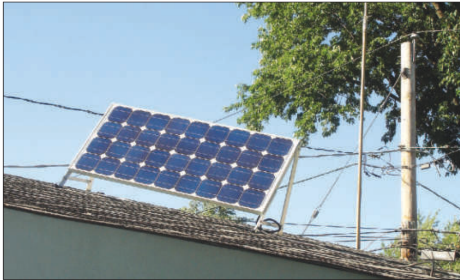
Figure 3 — The solar panel mounted on the garage roof. The odd looking angle is to optimize sun radiation capture, but also helps keep a low profile to minimize both wind resistance and neighbor annoyance.
