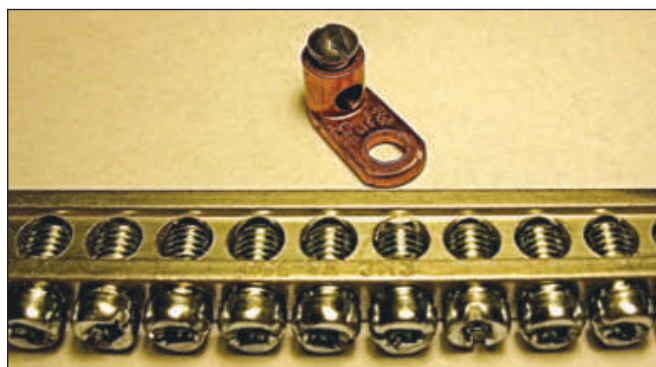
Figure 5 — The bus bar and the copper terminal lug.
