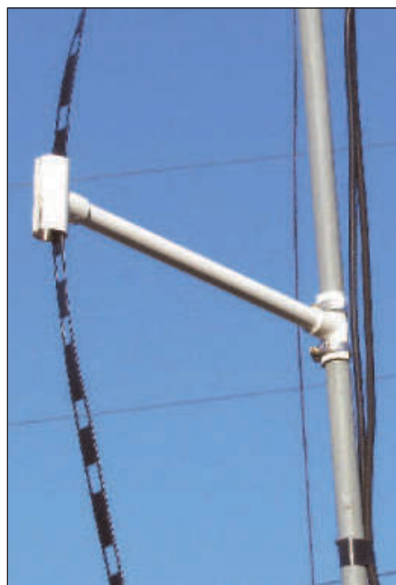
Figure 2 — Here is the PVC standoff holding the ladder line away from the metal mast. Note the modified T connector that is held to the mast using hose clamps.
