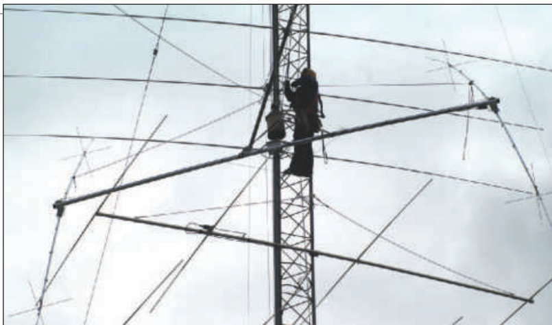
Andrew Toth guides the 40 meter beam into place as W1AW Station Manager Joe Carcia, NJ1Q, and Matt Strelow, KC1XX guide it up the tower from the ground.
