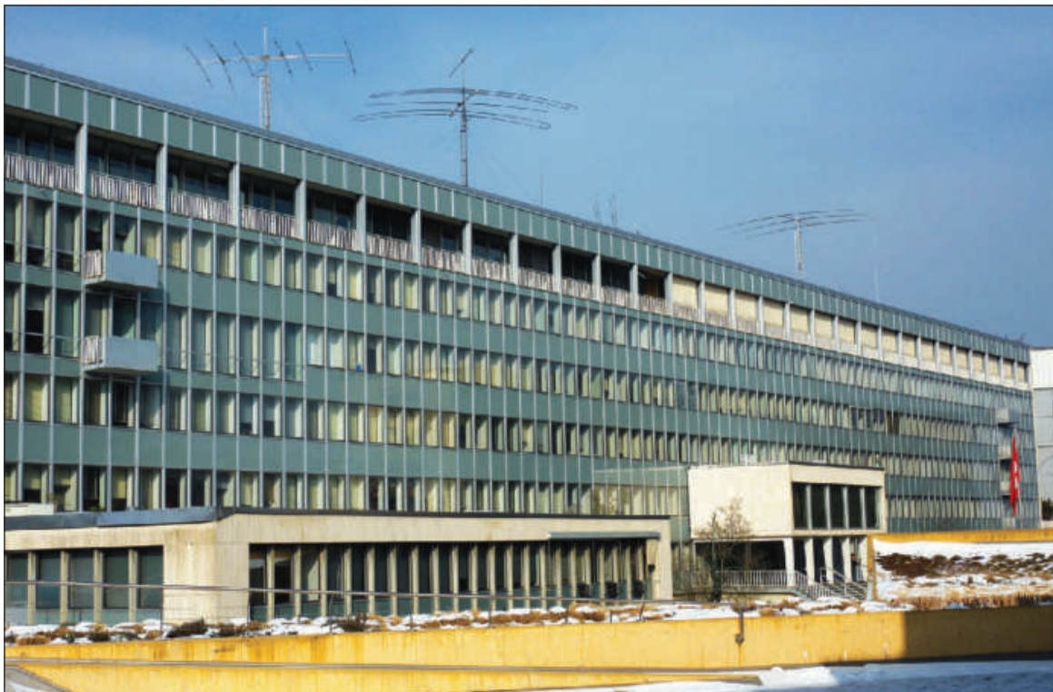
The antennas of International Amateur Radio Club station 4U1ITU are located on the roof of one of the ITU's three buildings. The special call sign 4U1WRC was used during the conference, reverting to 4U1ITU for the ARRL CW DX Contest the following weekend. [Ole Garpestad, LA2RR, photo]
