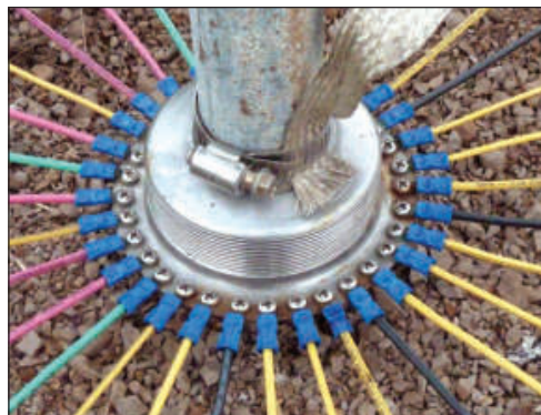
Figure 1 — The sink strainer radial ring, hose clamp and braid installed at the antenna base. The ground braid connects to the coax shield. [Ray DuFlon, KE6PXU, photo]
