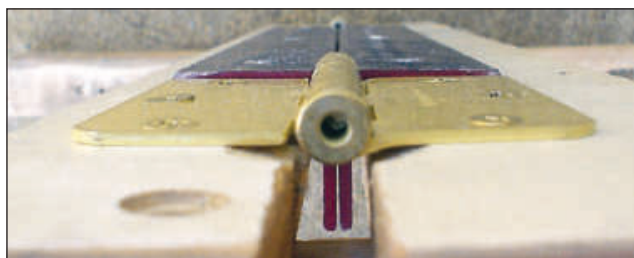
Figure 1 — For proper operation, it is important that the hinges be aligned as shown.
