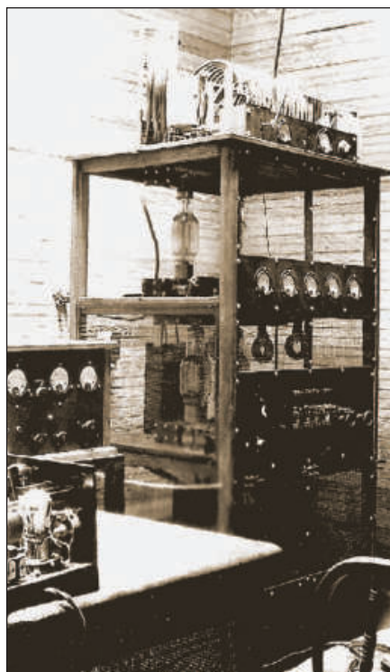
Figure 2 — While a graduate student at the University of Arkansas in the 1920s, Barton designed and constructed this 500 W transmitter. It would become the world's first high-level class B plate modulated rig. [James O'Neal, K4XAR, photo]
