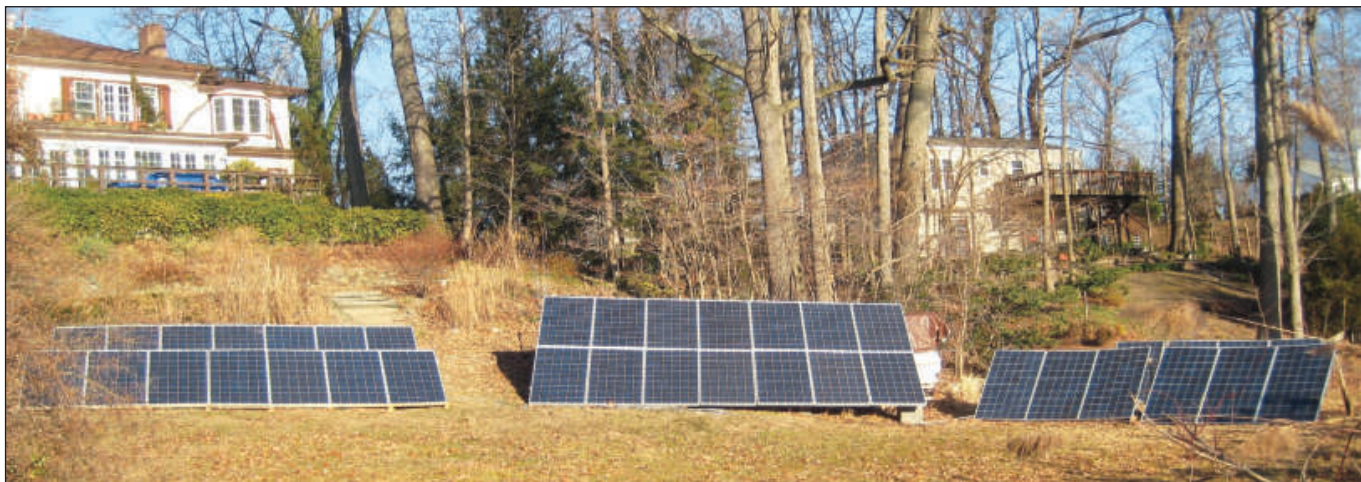
Figure 4 — My home 8 kW grid-tie solar system also provides emergency power when the grid goes down by connecting to switching power supplies.
