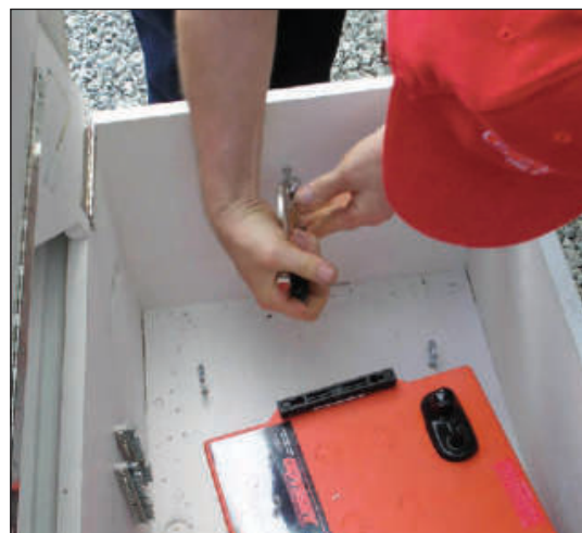
Figure 3 — Installing battery hold downs and wiring blocks.
