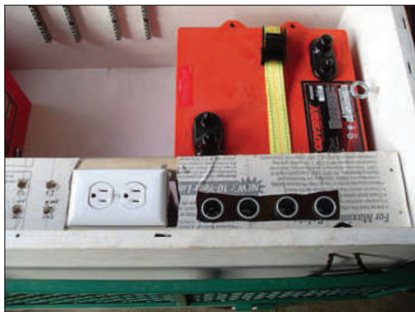
Figure 7 — Control panel with power outlets. See text regarding lack of GFCI.
