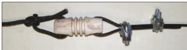
Figure 6 — End insulator detail. The same type of clamps are used as those in the center. These make length adjustment easy.
