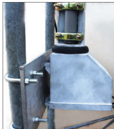
Figure 4 — This arrangement of the rotator and mounting plate lines up with the mast bushing on a Rohn 25 tower top section. [Jack Morgan, KF6T, photo]
