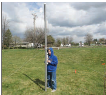
Figure 8 — Partially constructed array during mast alignment.
