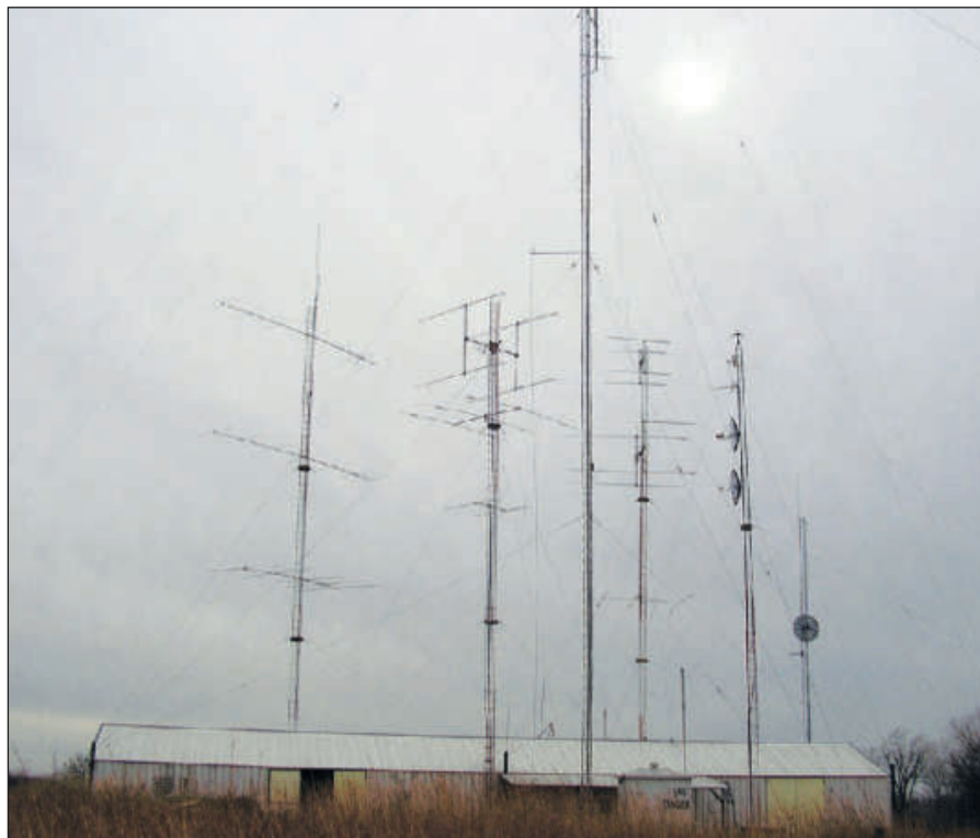
These towers full of antennas kept Gary Gerber, KB0HH and his ops on the bands and loud, too! Gary and his “Bunkhouse crew” earned third place in the Multioperator category from his EM06 QTH. [Photo courtesy Gary Gerber, KB0HH]
