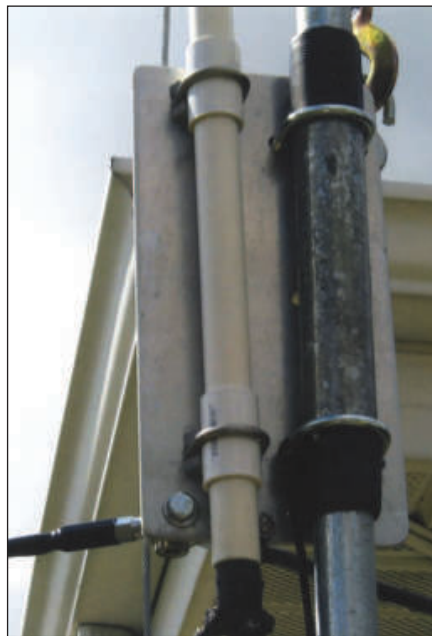
Figure 3 — View of the trolley on the 10 foot length of the 1-1/4 inch galvanized steel pipe. This trolley is the means by which the antenna slides up and down the 10 foot pole.
