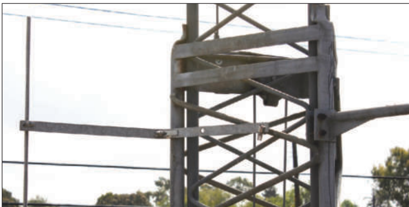
Figure 3 — Upper bracket and gamma rod.
