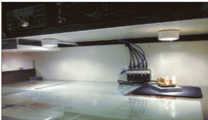
Figure 3 — A 1 inch opening that runs along the back of the cubby allows for passing wire and cable through from the operating area. Also visible are the halogen lights and the white enamel paint used to brighten the workspace.
