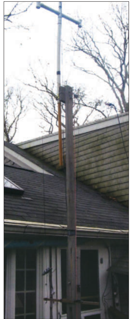
Figure 4 — Close up of the upper mast section showing the antenna attachment methods employed.
