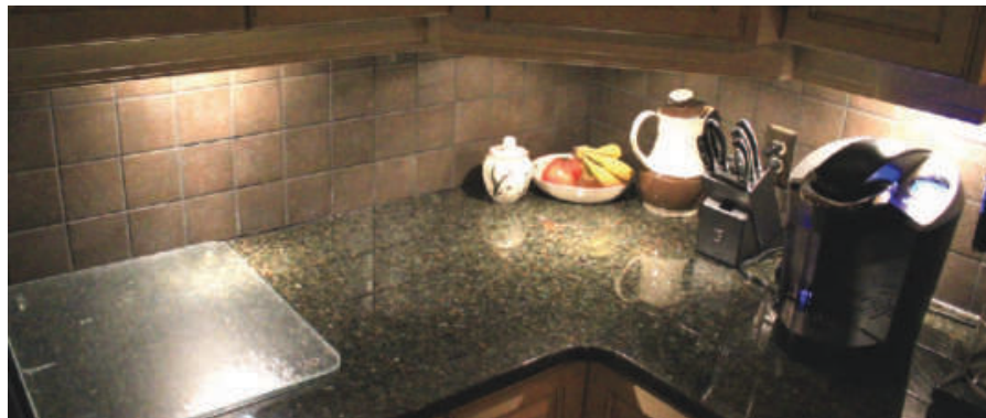
Figure 1 — Low voltage, high intensity halogen lamps were installed under the kitchen cabinets to illuminate the counter top.
