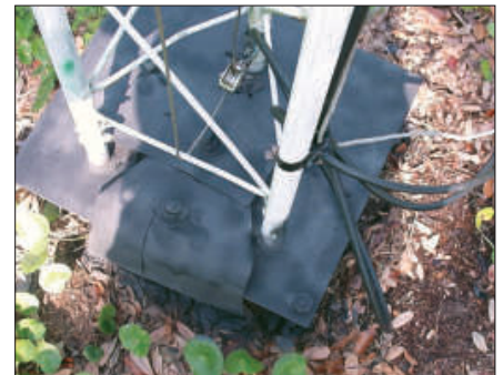
Figure 3 — This pulley added to the bottom of the tower redirects the cable toward the post mounted winch. In this view the cable is not in use, runs out of the tower and turns upward and out of the way. [Pat Hamel, W5THT, photo]
