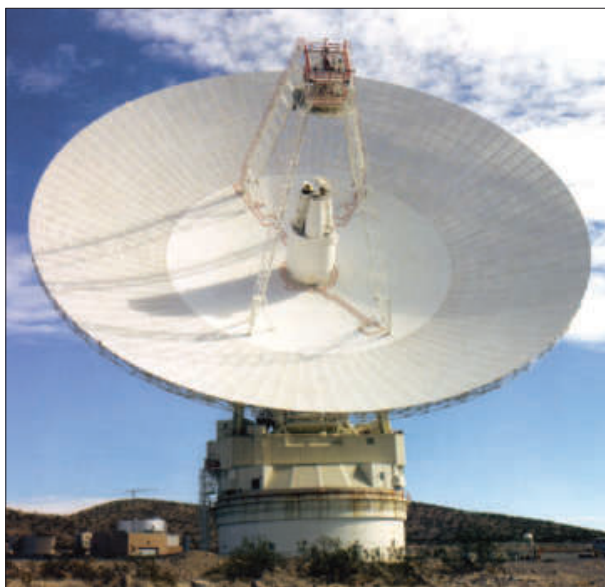
The prime antenna used for communicating with the Cassini spacecraft is a 230 foot wide parabolic dish antenna of the type pictured here at NASA's Goldstone site in California's Mojave Desert. The two other similarly equipped sites are in Australia and Spain.
