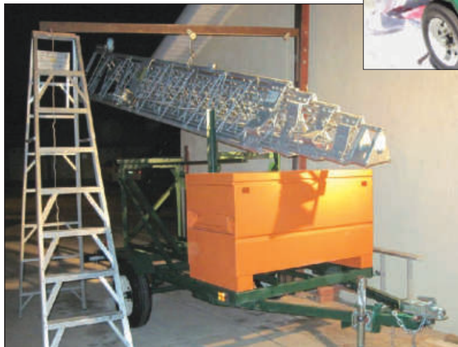
This is the hoist setup I used to place the tower onto the trailer.
