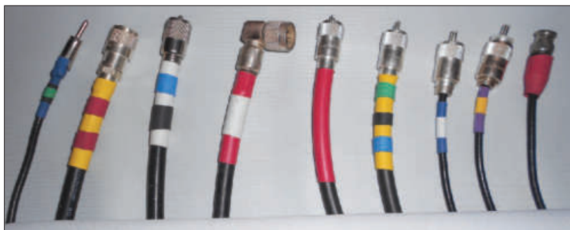
Figure 6 — Colored heat shrink applied to the ends of cables can be used to indicate length or application at a glance. [Walter Martin, KB5HOV, photo]
