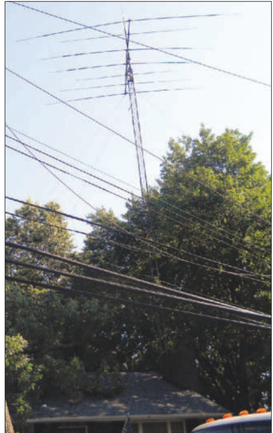
When I walked outside after the storm and saw my tower, it was obvious that something was very wrong!
