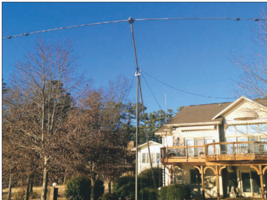
Figure 7 — Rotating the antenna upward using a surplus mast push stick. Note that the wire dipole for 80 meters is not yet connected.
