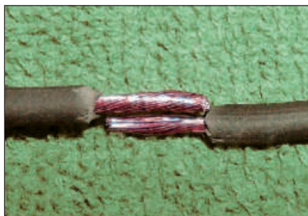
Figure 2 — To prepare a parallel splice, strip the ends of the wire and position them alongside each other. [Frank Ingle, KG4CQK, photo]
