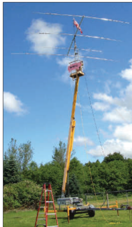
The flag is flying, and so are the pigs, atop one of the makeshift towers at the site of the Stanwood Camano ARC, W7PIG, near Stanwood, WA.
